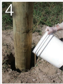
4 Pour mixture into prepared hole with pole
