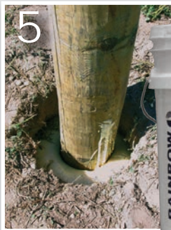
5 Let sit for 30 minutes; hardware is ready to be strung
