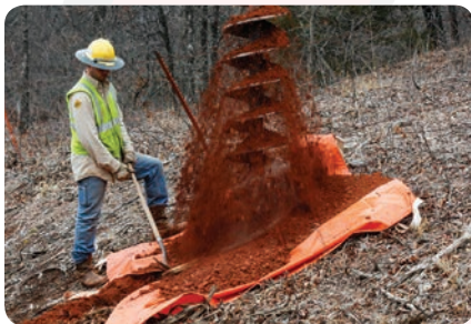
DirtBall in Action Installing a Utility Pole
