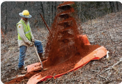
DirtBall in Action Installing a Utility Pole
